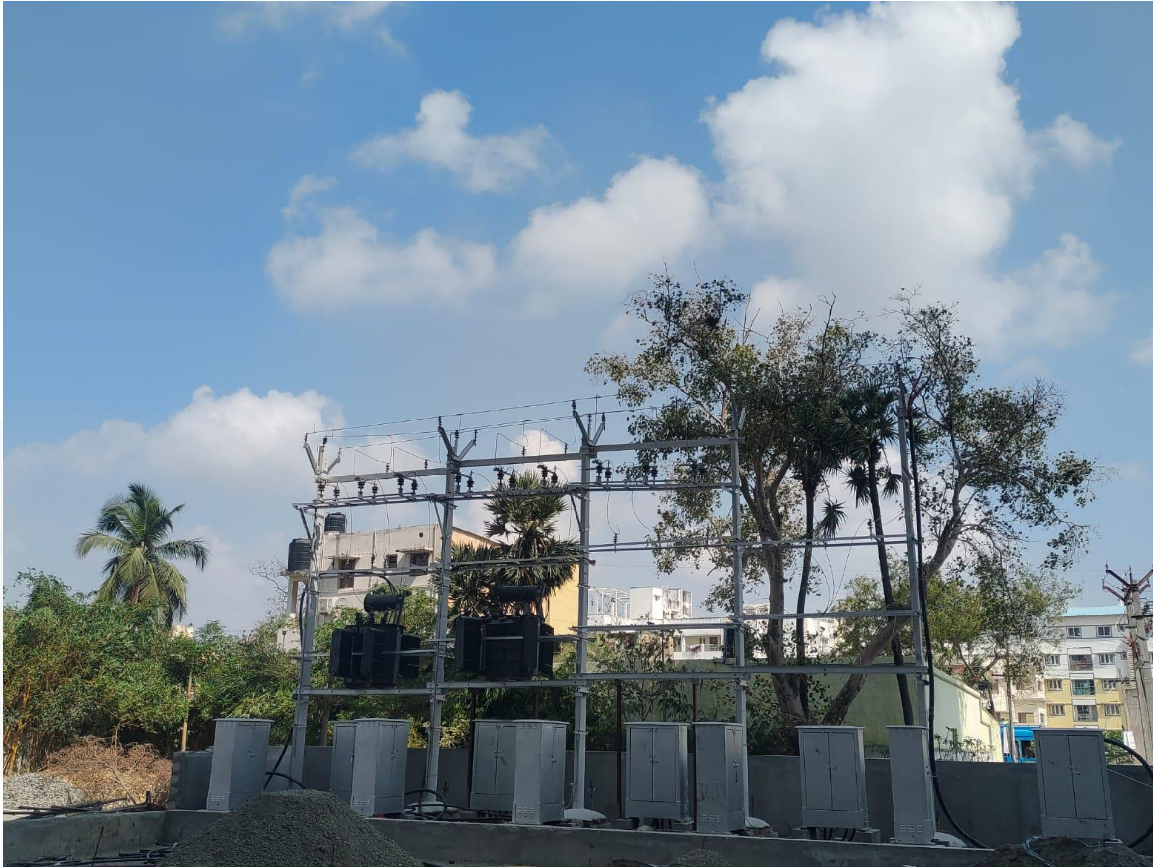
Transformer Erection Work In Progress
