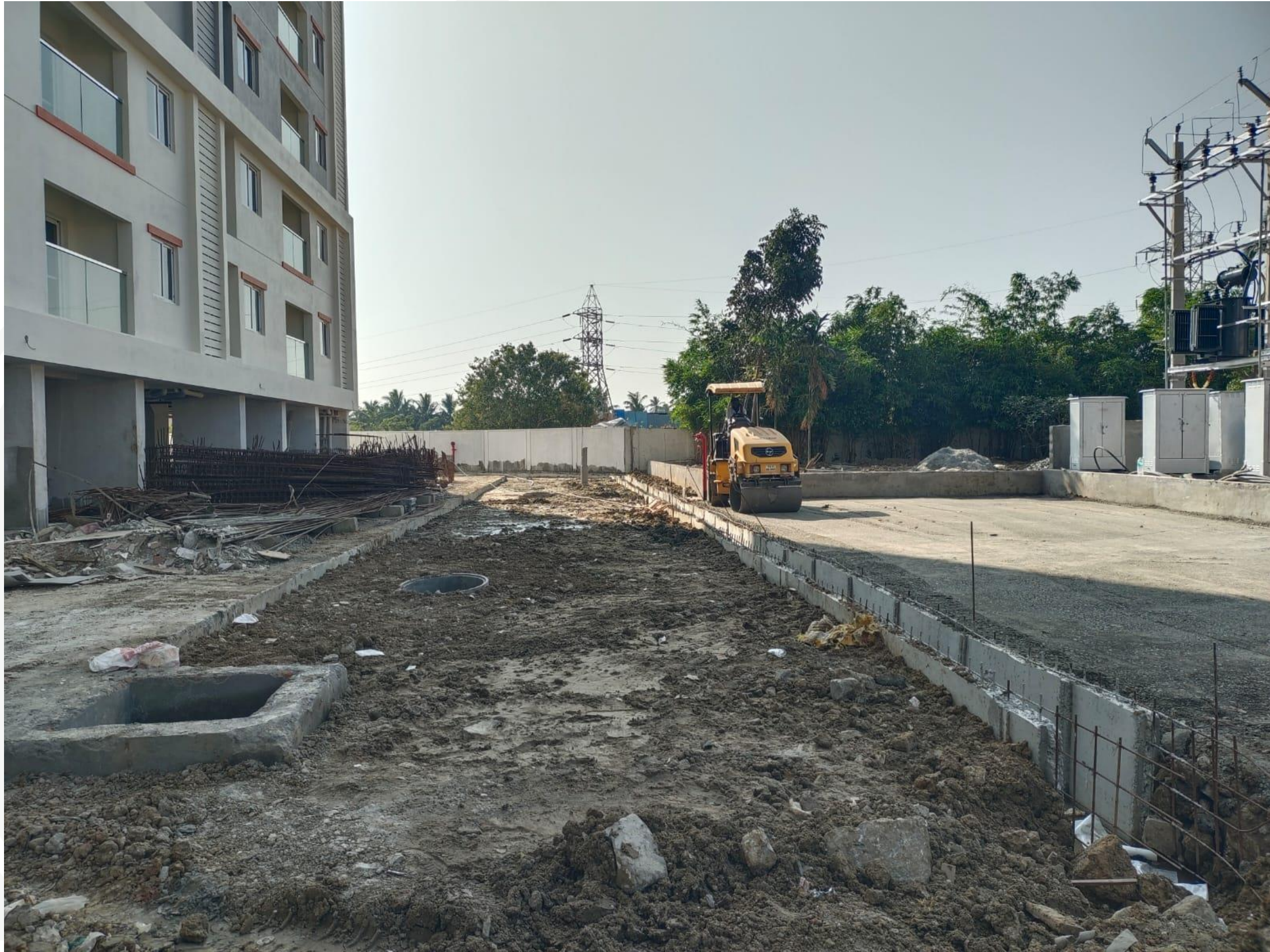
External Storm Water Drain Work In Progress
