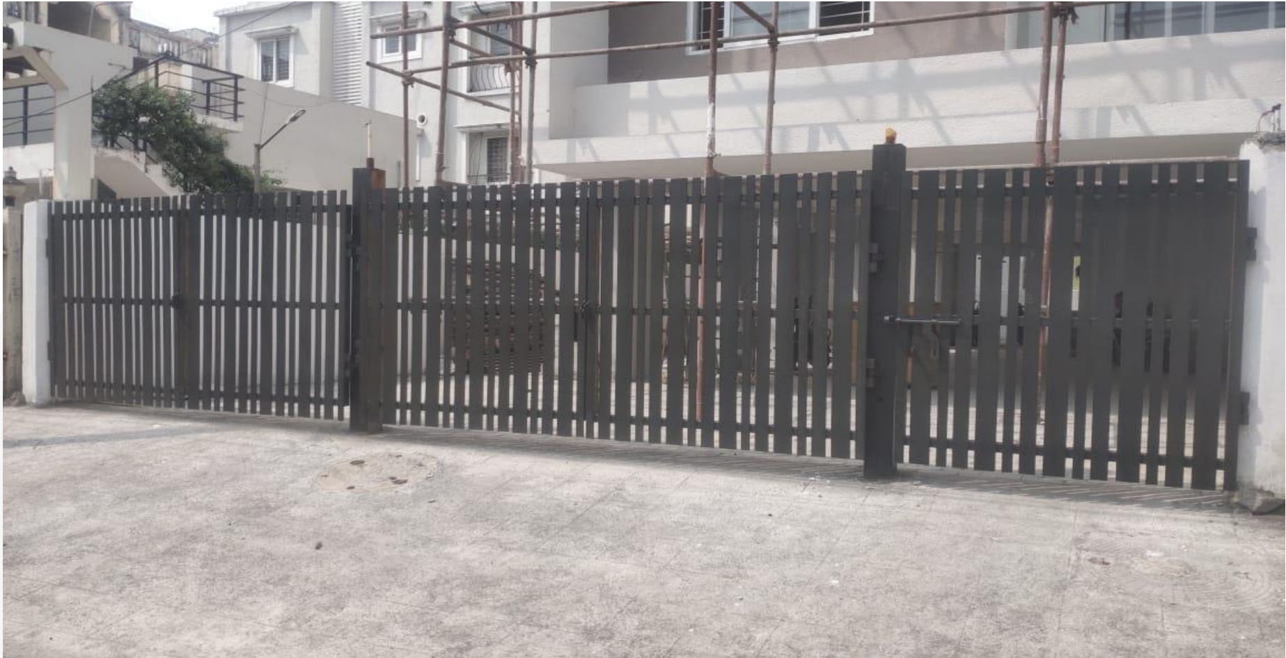
Gate painting work
