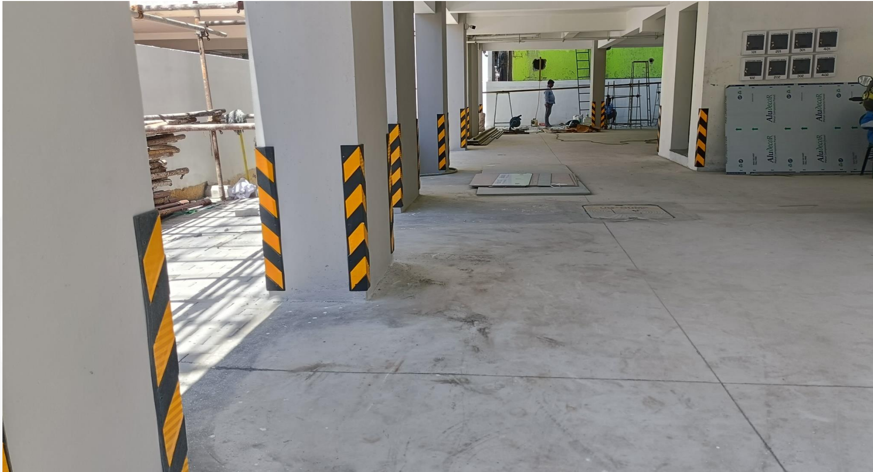
Column guard fixing work completed
