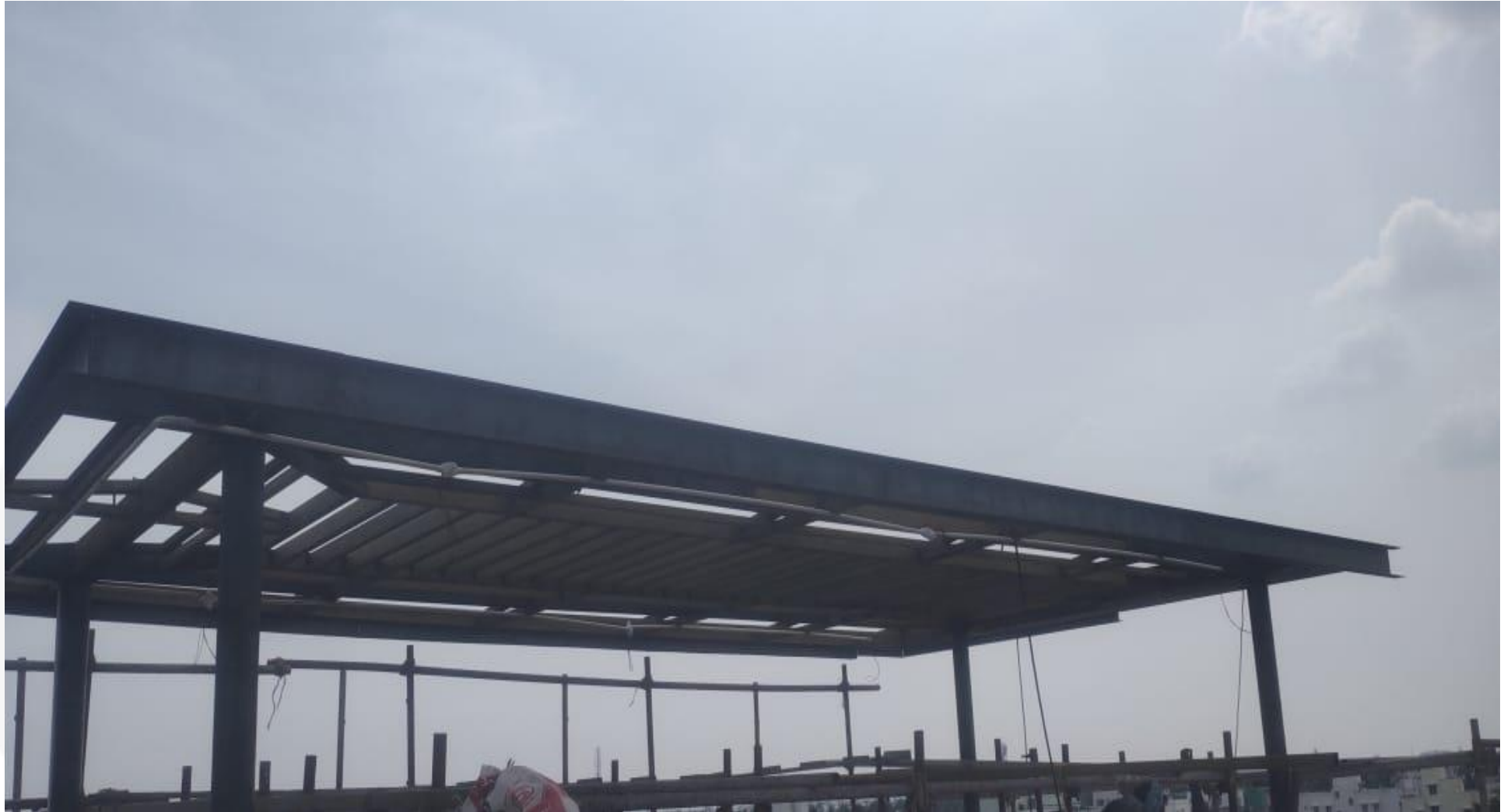
Terrace pergola MS painting work completed
