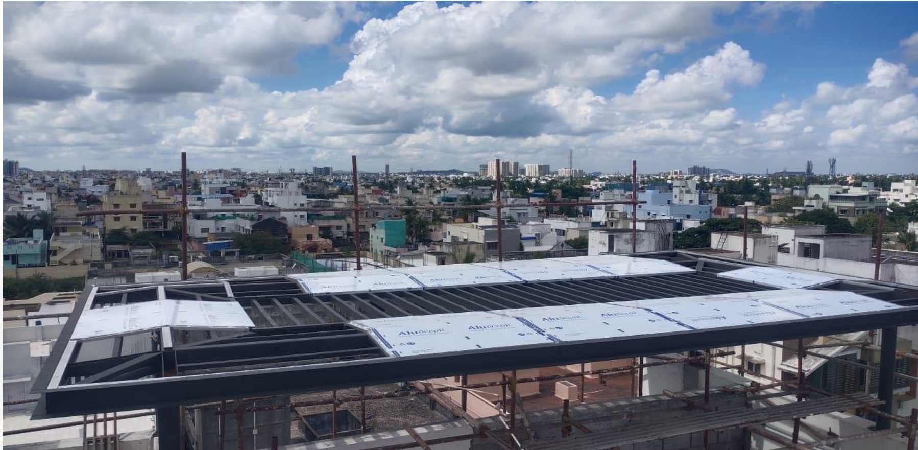
Terrace Pergola ACP cladding work in progress
