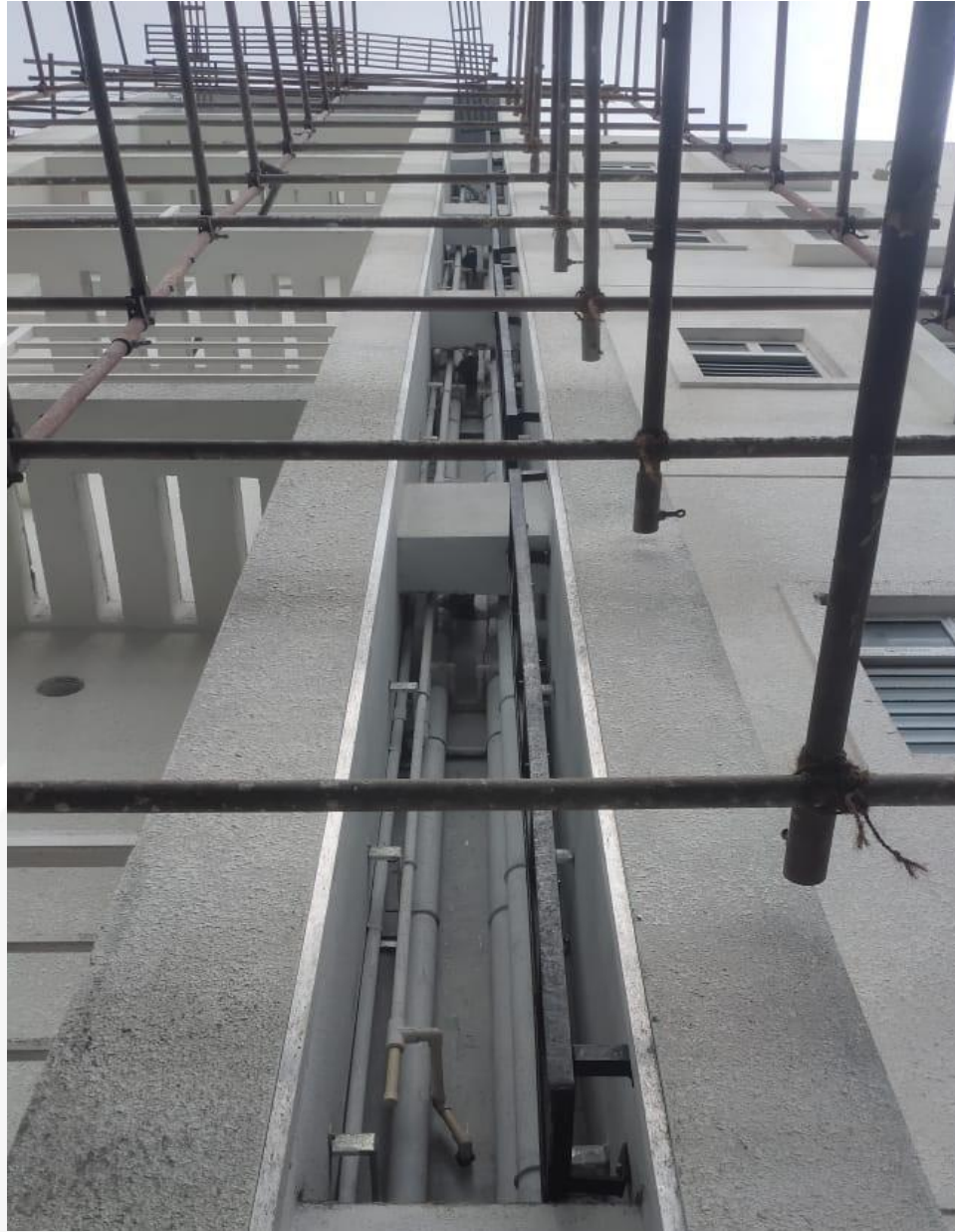
East side external AC service ladder work completed
