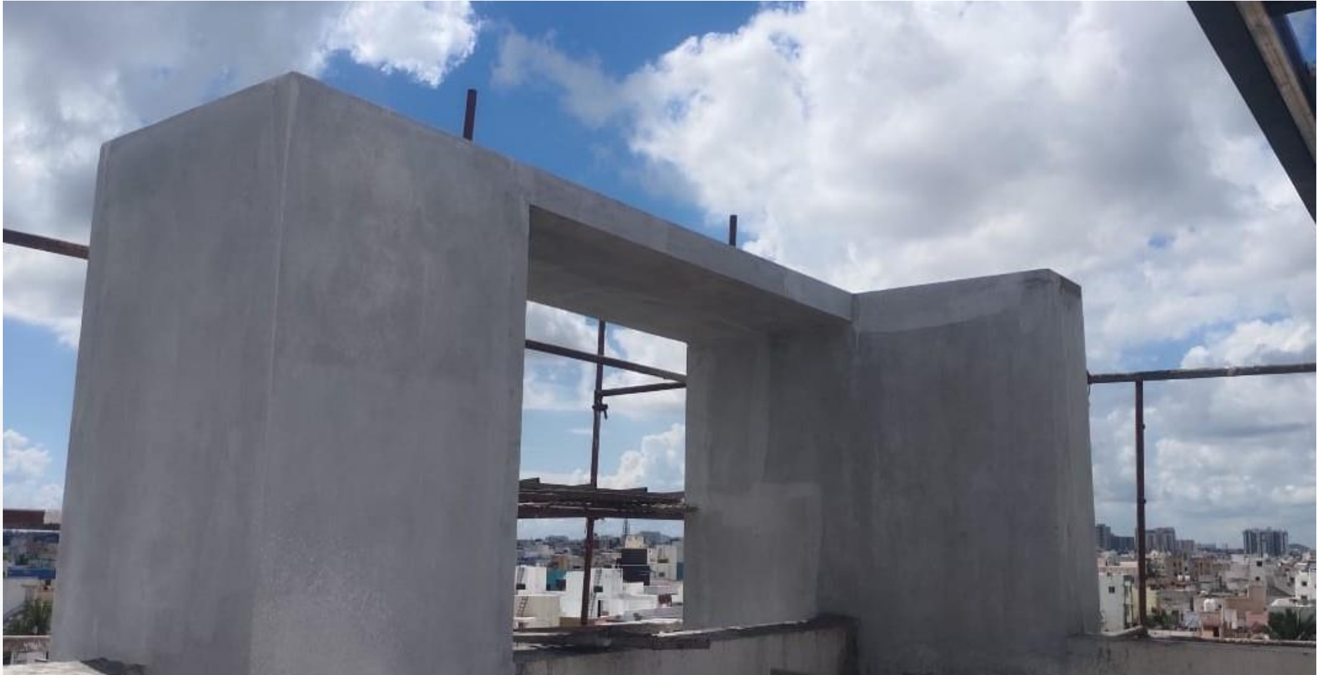
Terrace Elevation slab work completed
