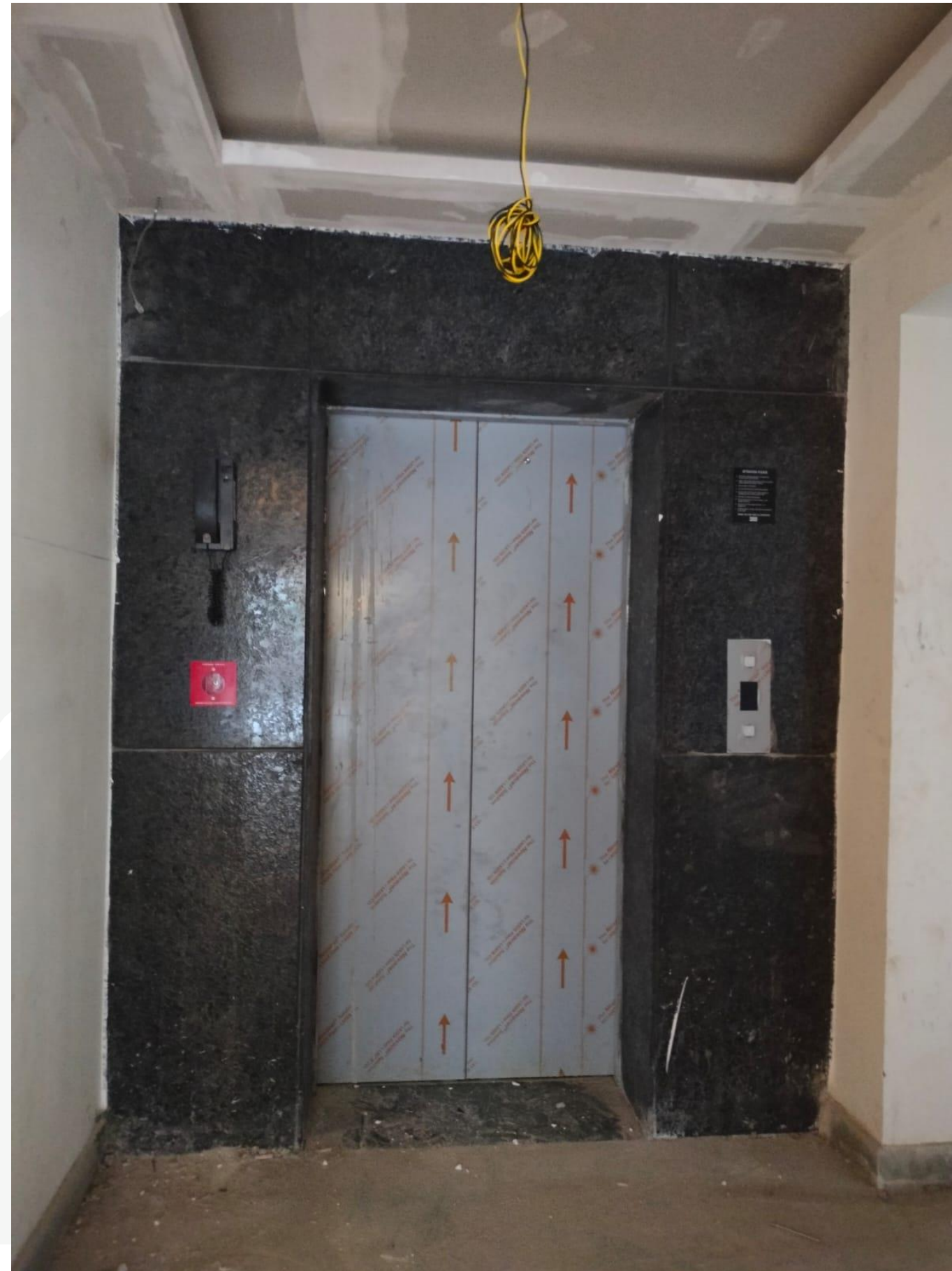
Lift -2 & 3 Erection Work In Progress ,
