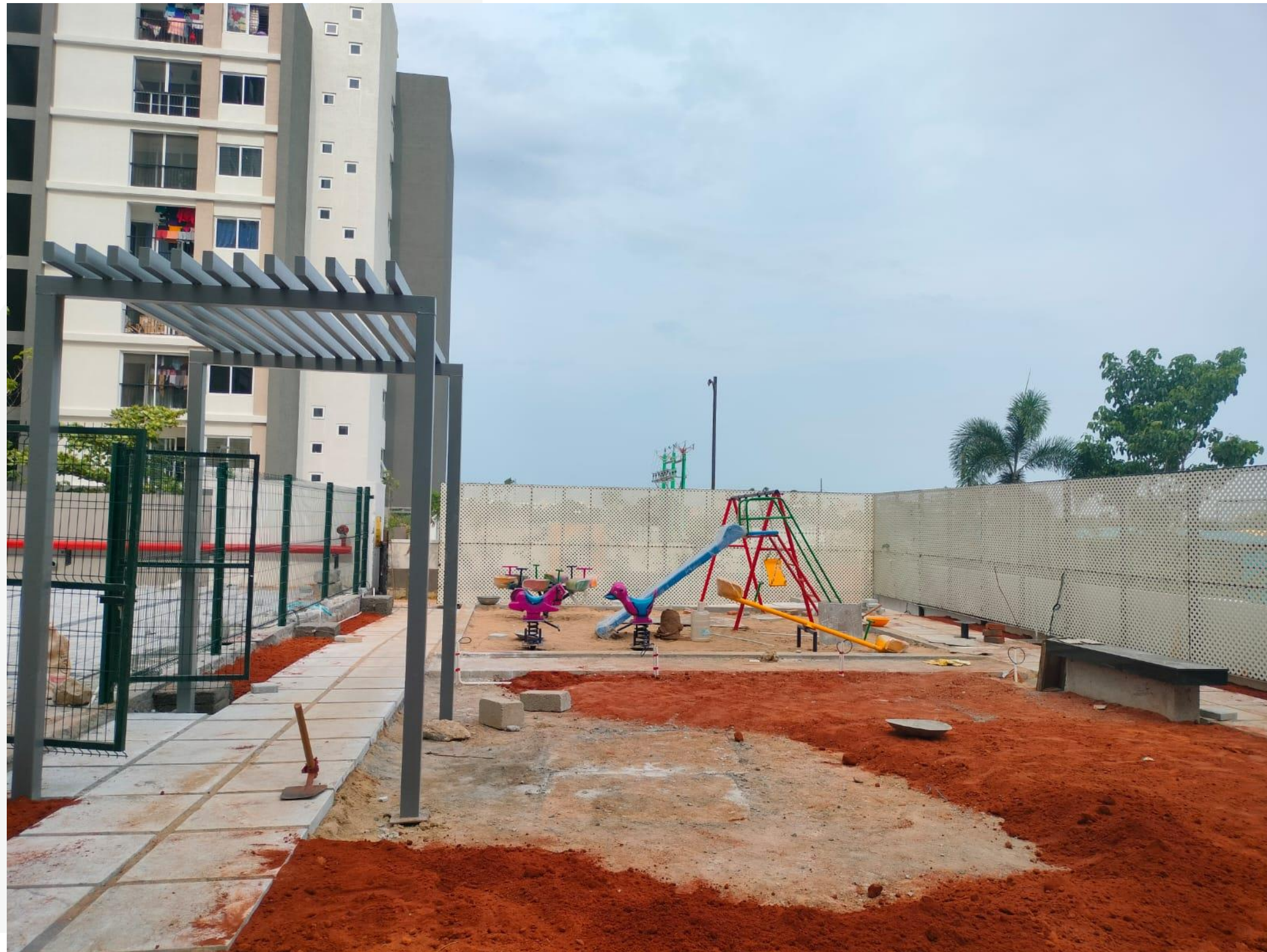
OSR Landscape Work In Progress
