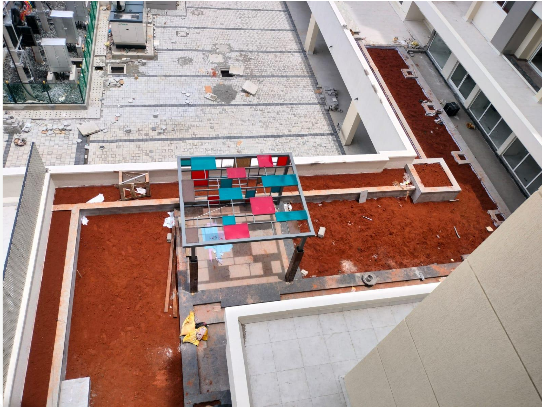
1 st Floor Amenities Hardscape Work in progress
