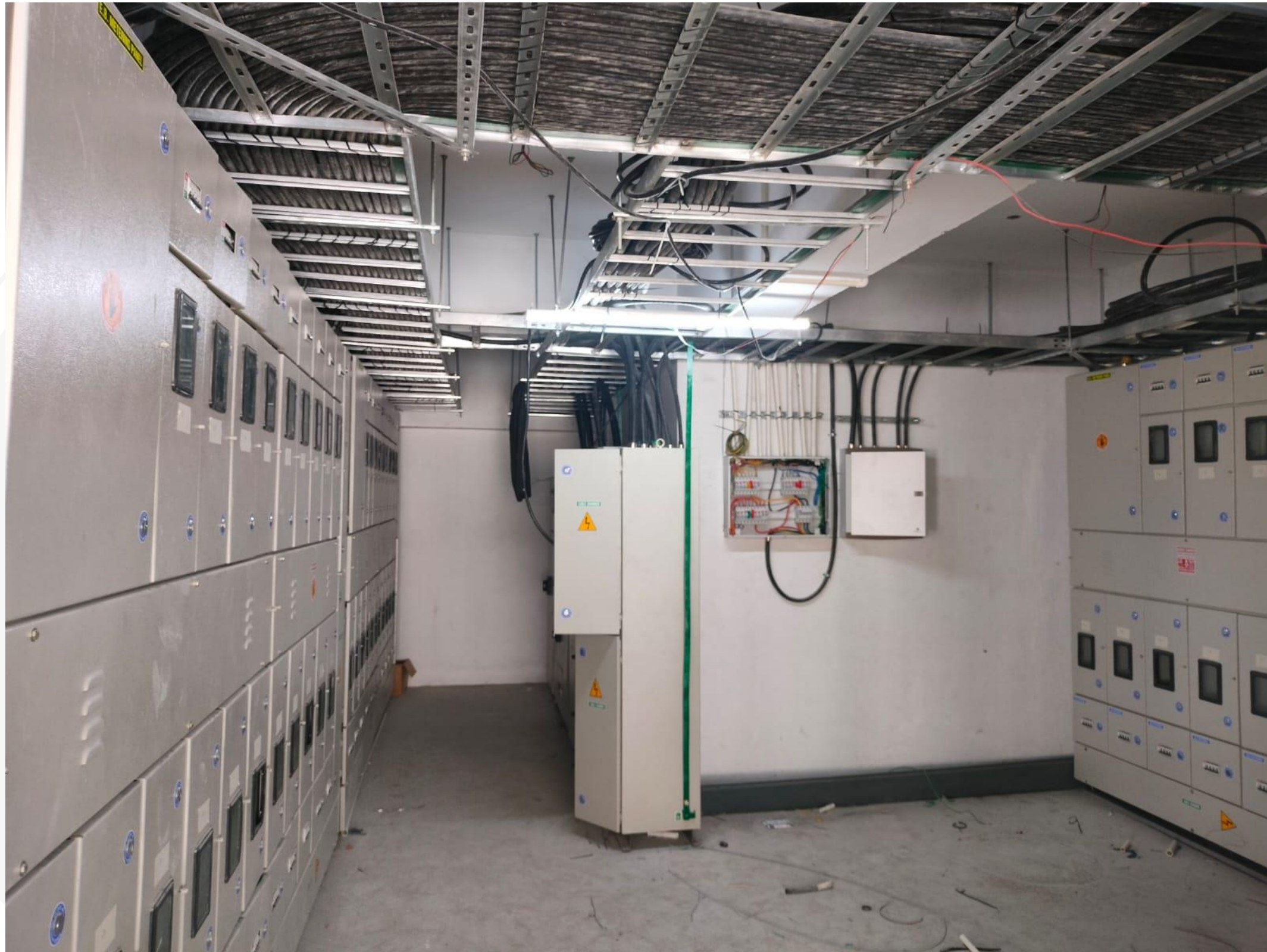
Electrical Room-1&2 Termination Work In Progress ,
