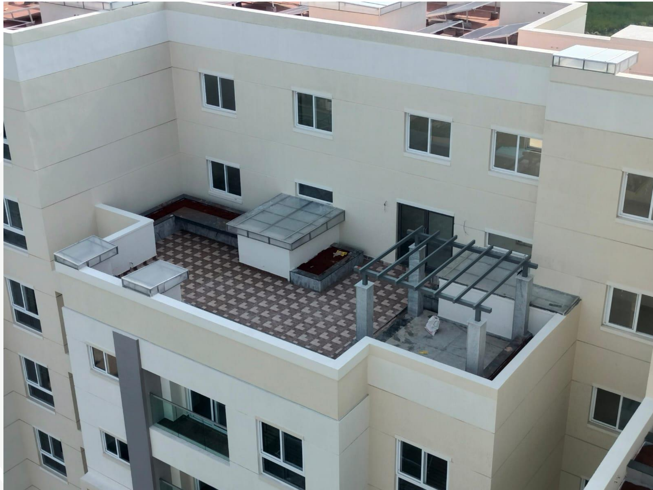
10 th Floor Level Low Terrace Hardscape Work In Progress
