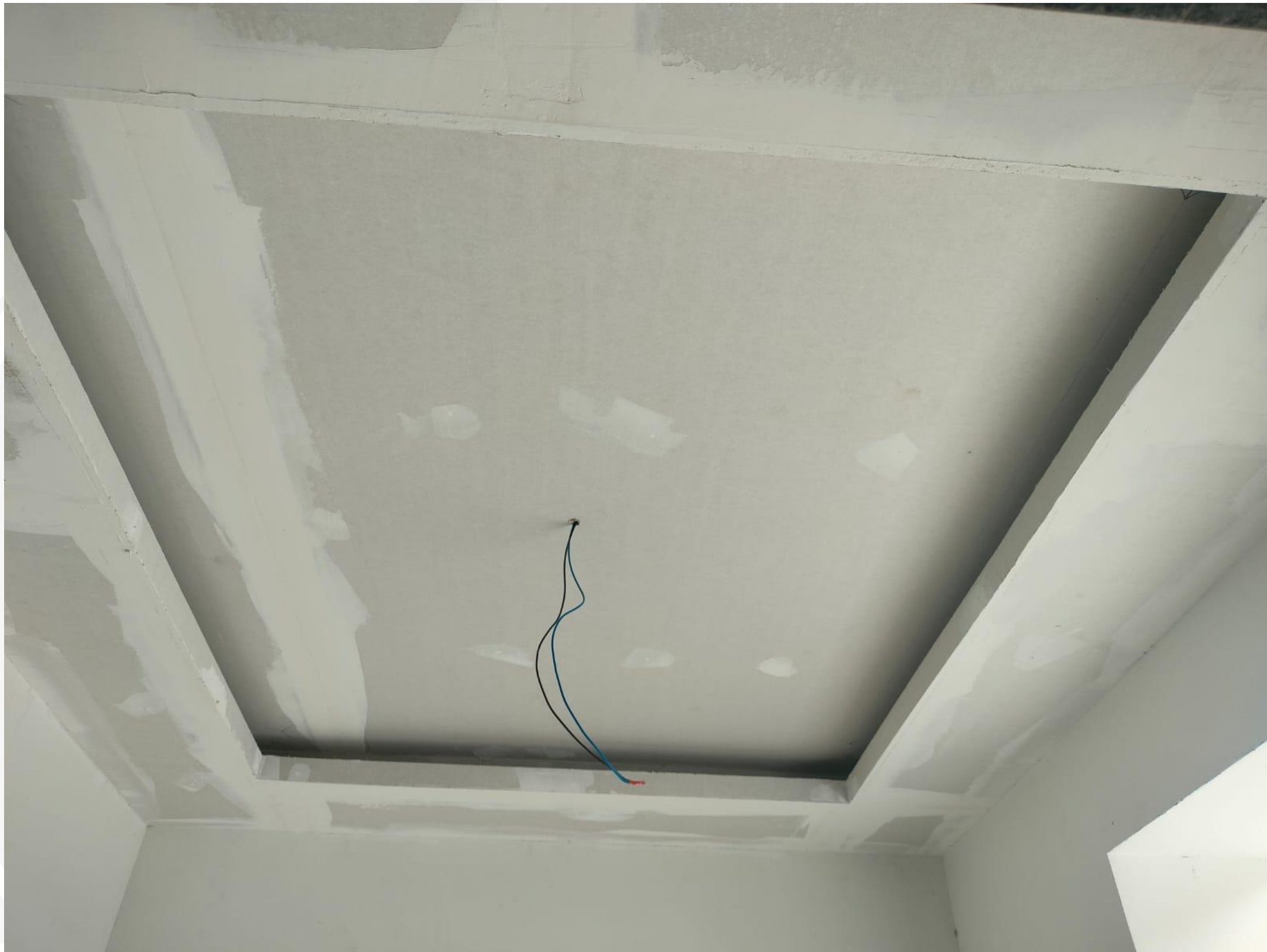
Stilt Floor Lift Lobby False Ceiling Work Completed
