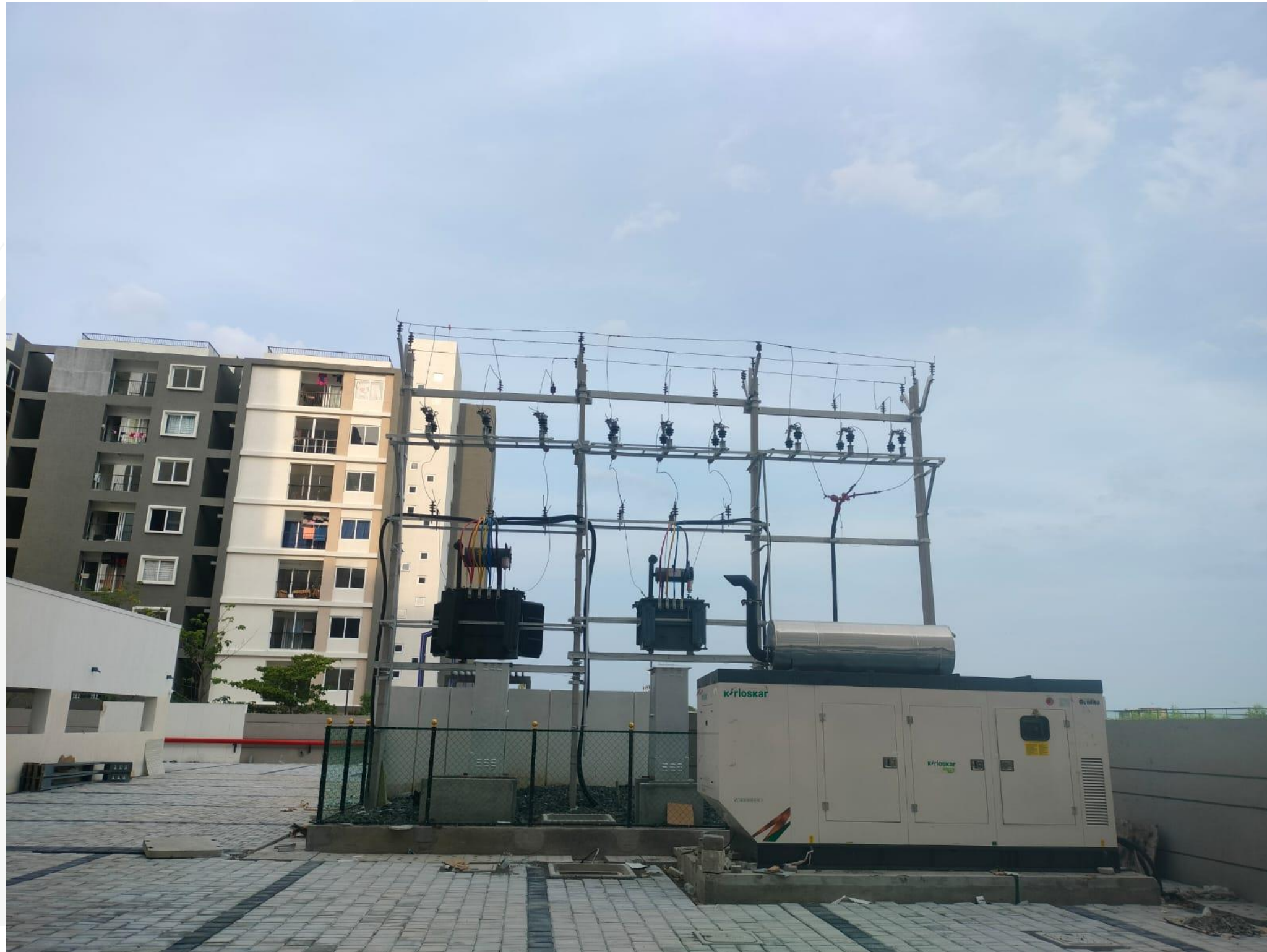
Transformer Erection Work Completed
