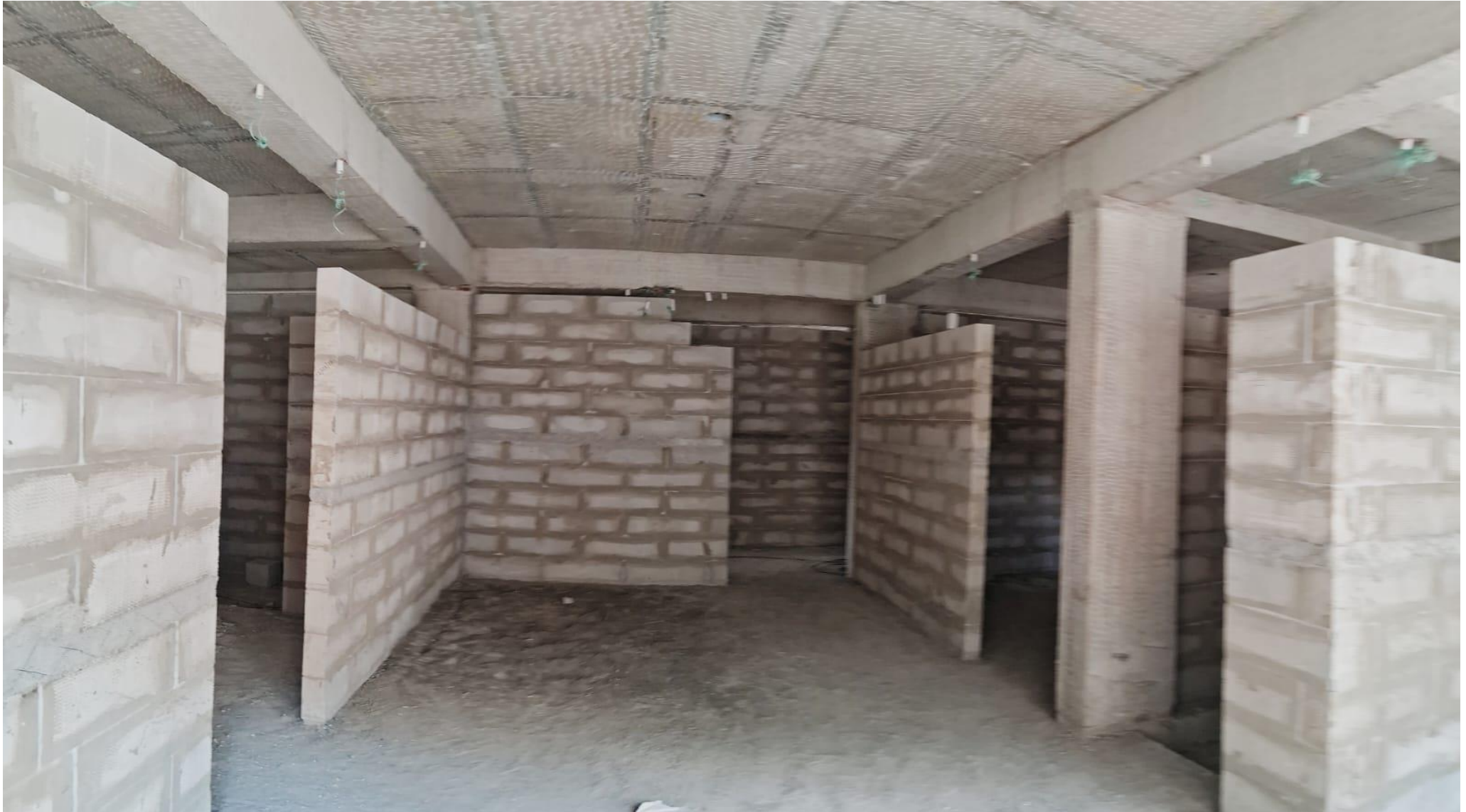
Second Floor AAC Block Work In Progress- Wing 3C
