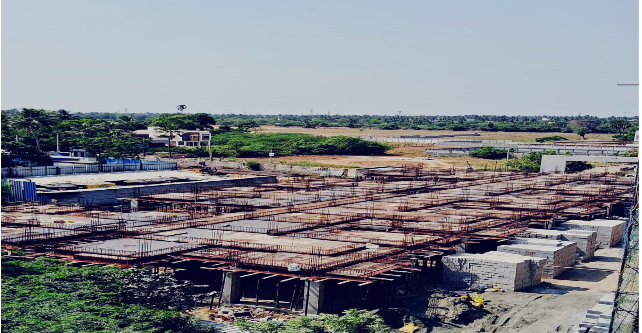
Stilt Floor Roof Work In Progress - Block 4
