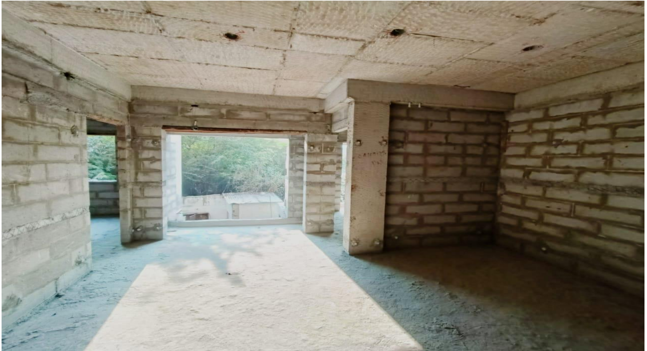
First Floor AAC Block Work Completed - Wing 3C
