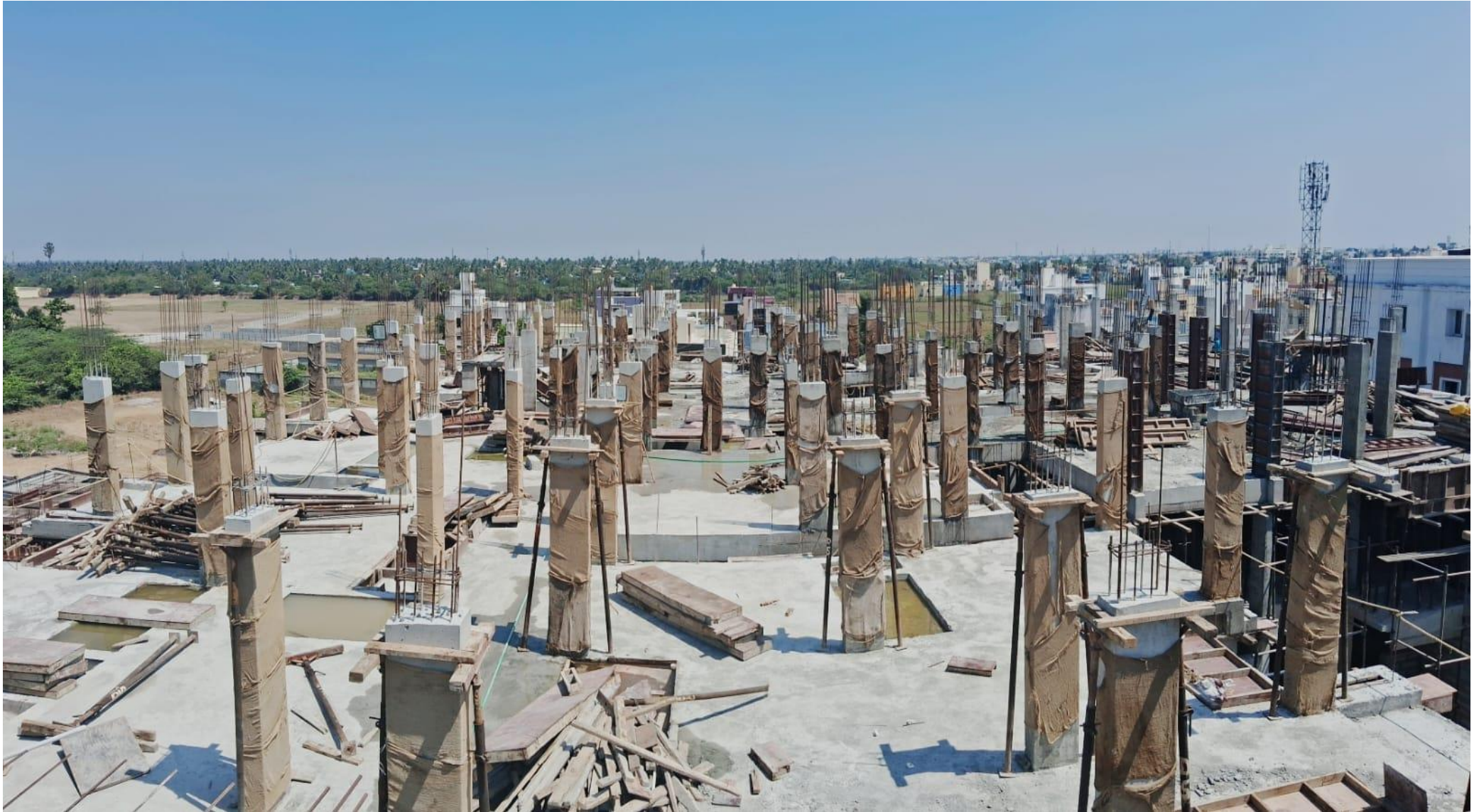
Fourth Floor Column Work Completed - Wing 3A & 3B
