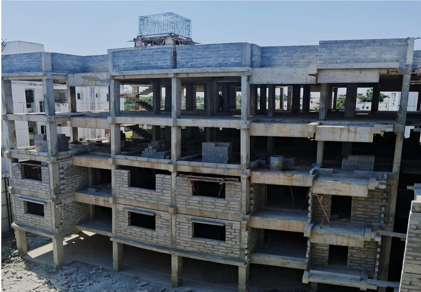
Wing 3E - Second Floor Block Work In Progress
