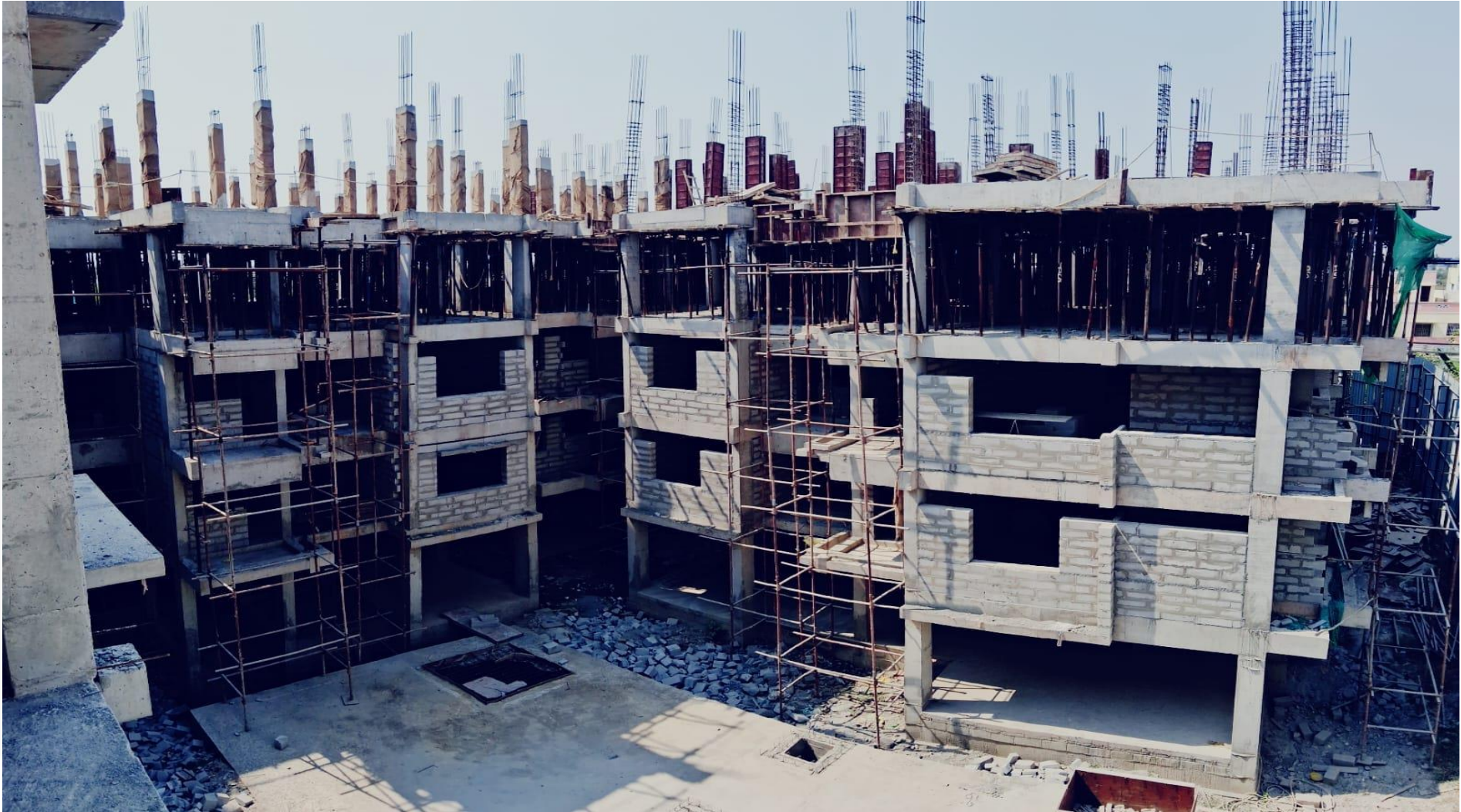
Wing 3A & 3B – First & Second Floor Block Work In Progress
