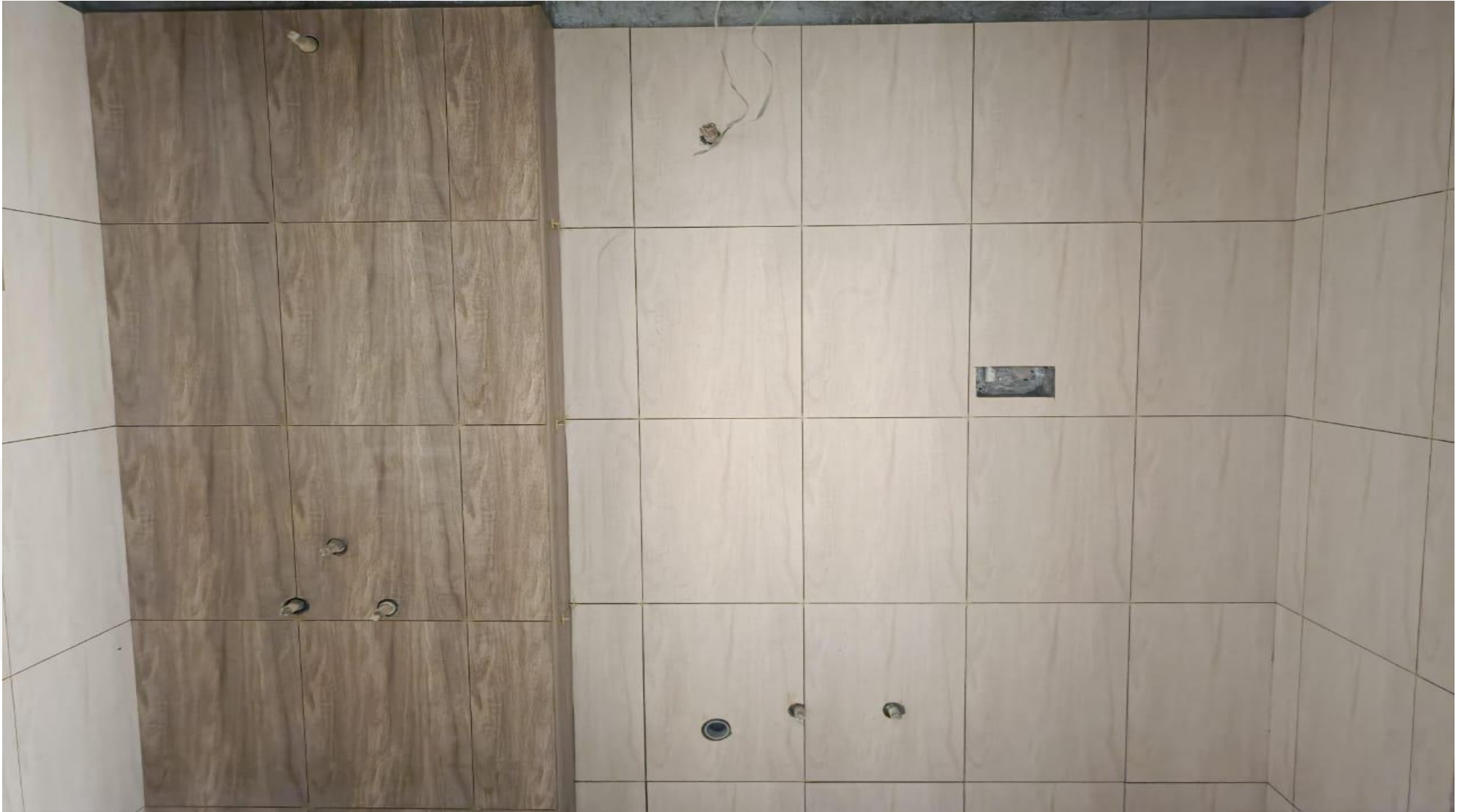
Wing 3D, 2 nd Floor - Toilet Tile Works in Progress
