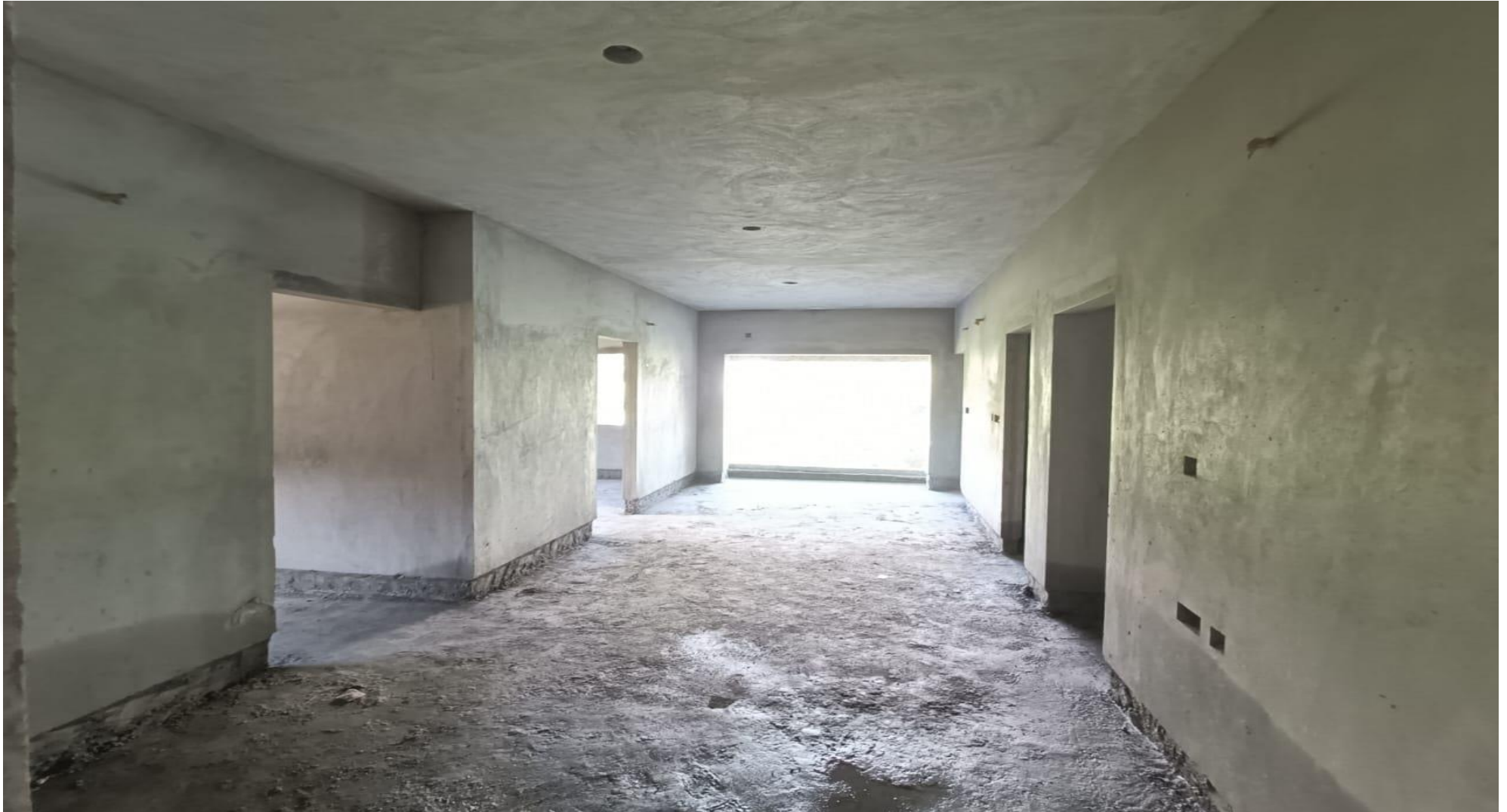
Wing 4A & 4B , 1 st Floor - Plastering Works Completed
