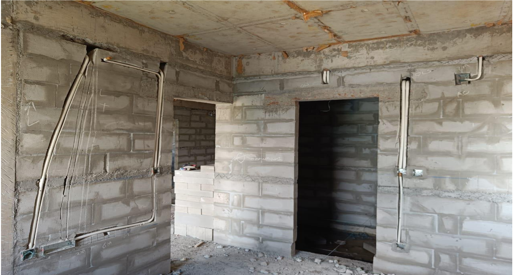
Wing 4A & 4B, 3 rd Floor - Electrical Wall Chasing work in progress
