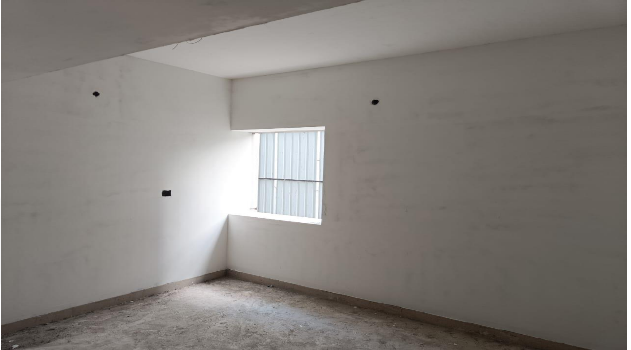
Wing 3D, 1 st Floor – Wall & Ceiling Putty Works in Progress
