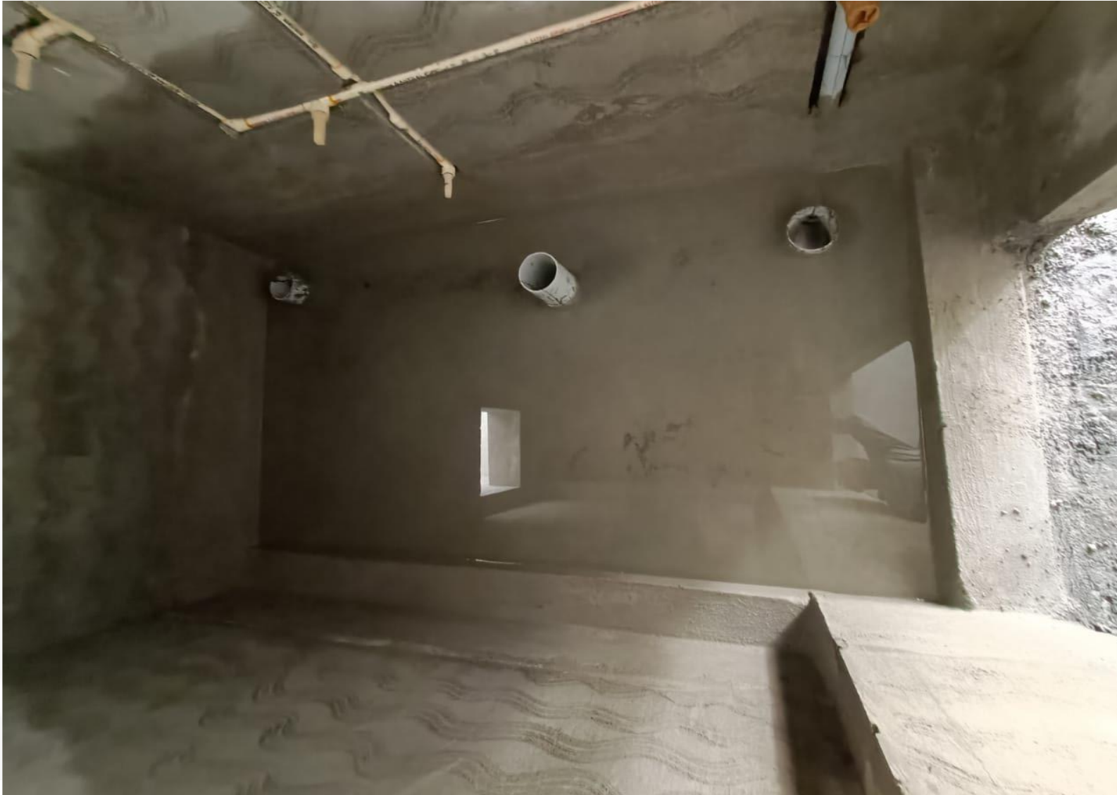
Wing 3C, 4 th Floor - Sunken Water Proofing Works in Progress
