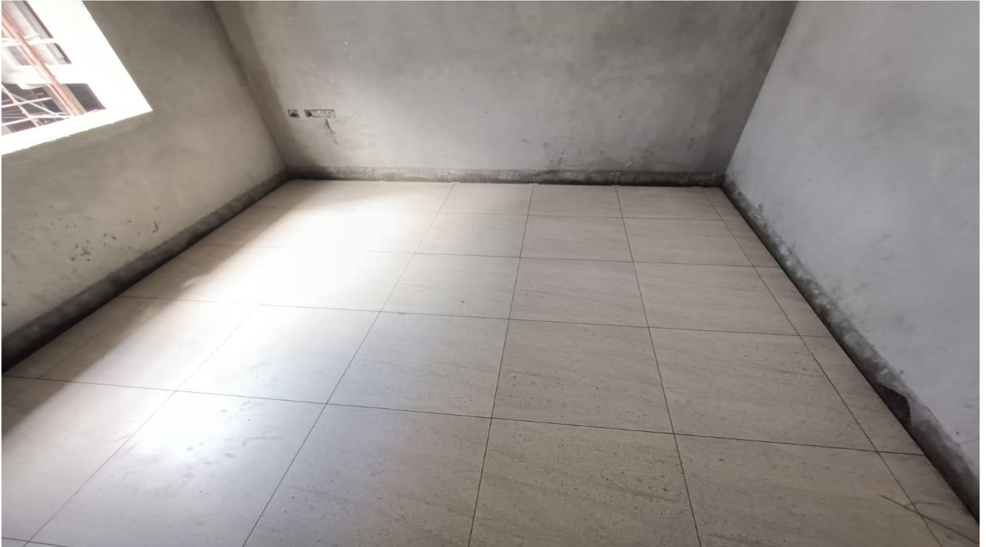
Wing 3D, 3 rd Floor - Tile Flooring Works in Progress
