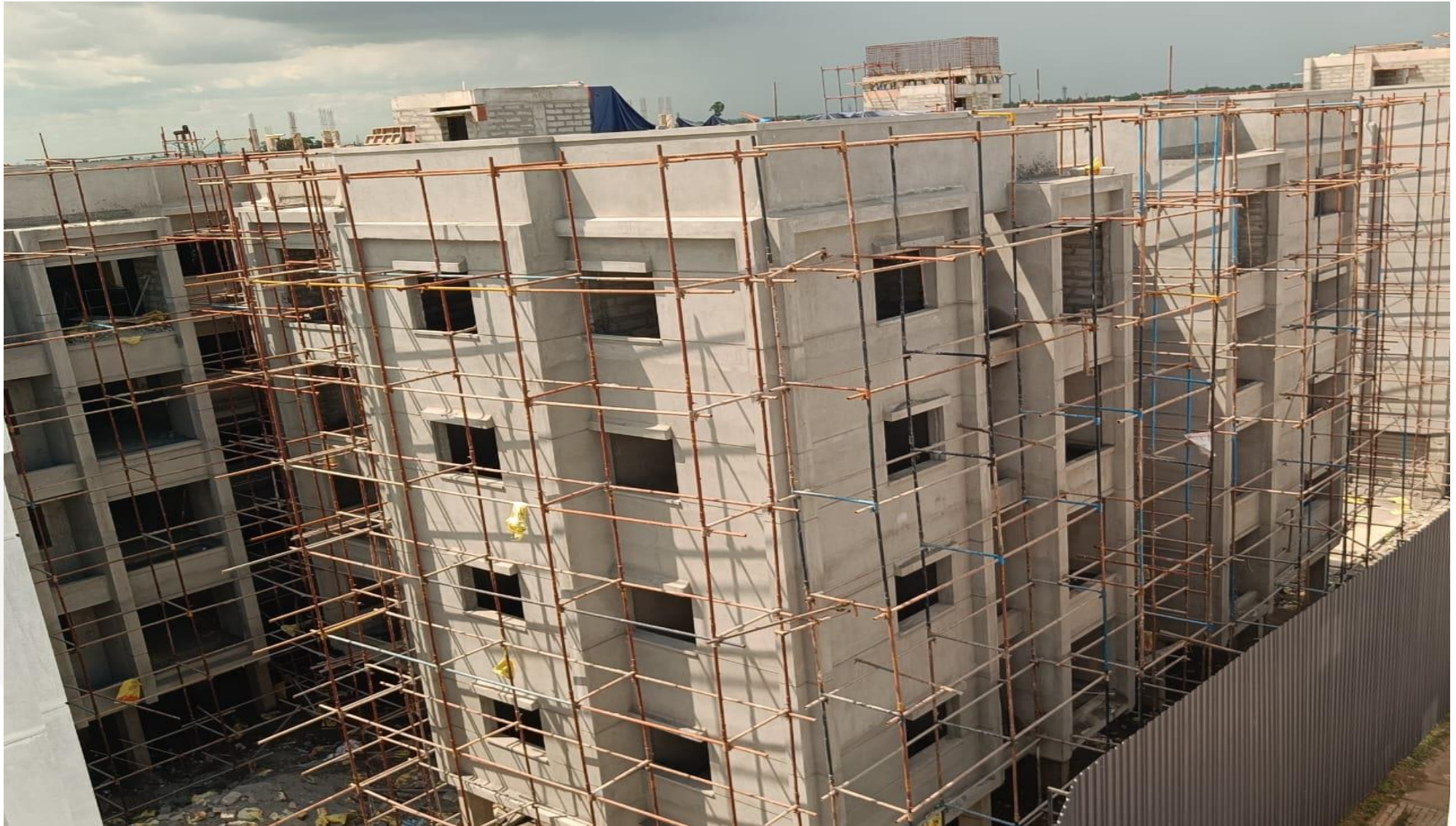
Wing 3C – South & East Elevation View
