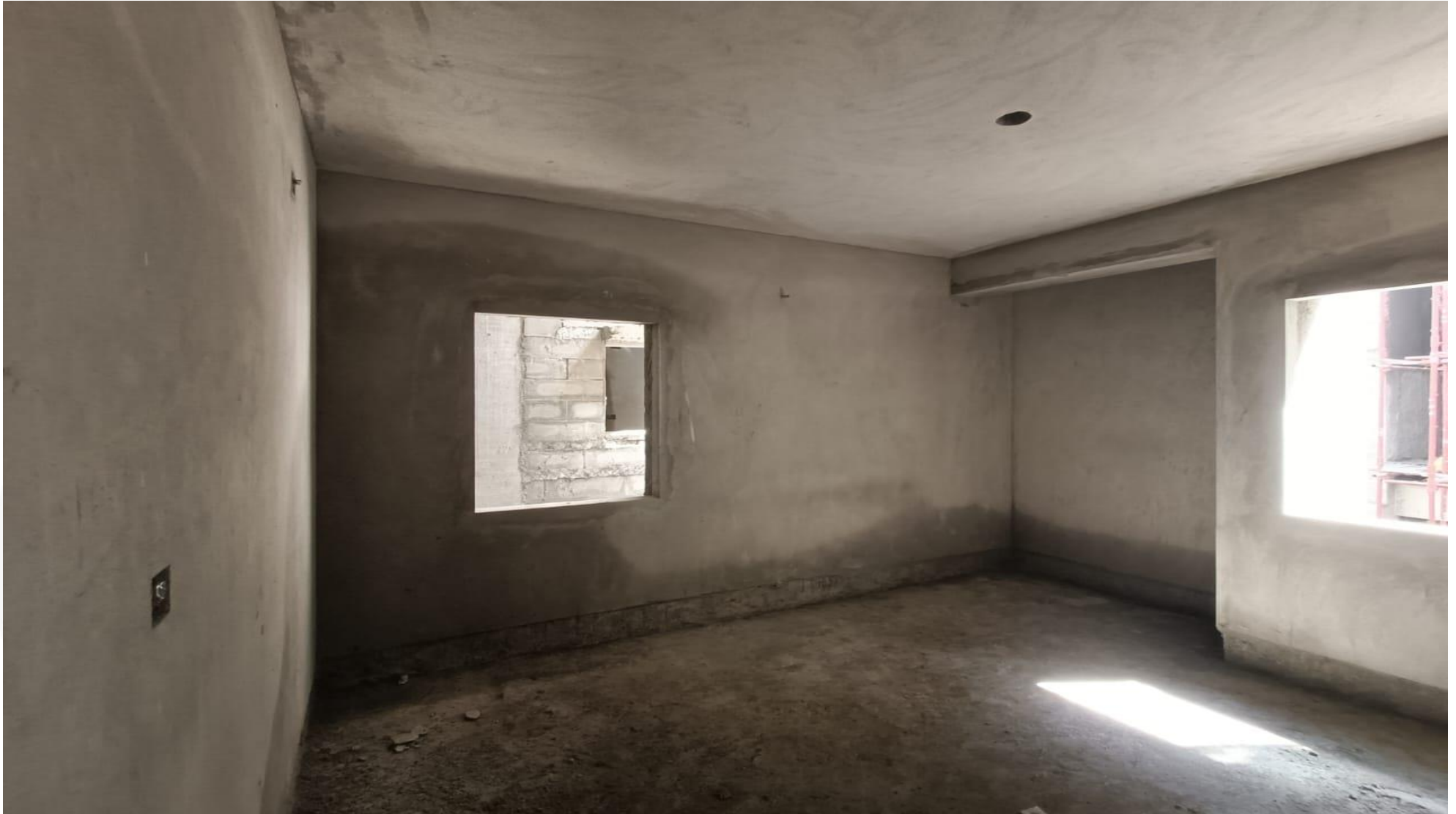
Wing 4A & 4B, 2 nd Floor - Plastering Works in Progress
