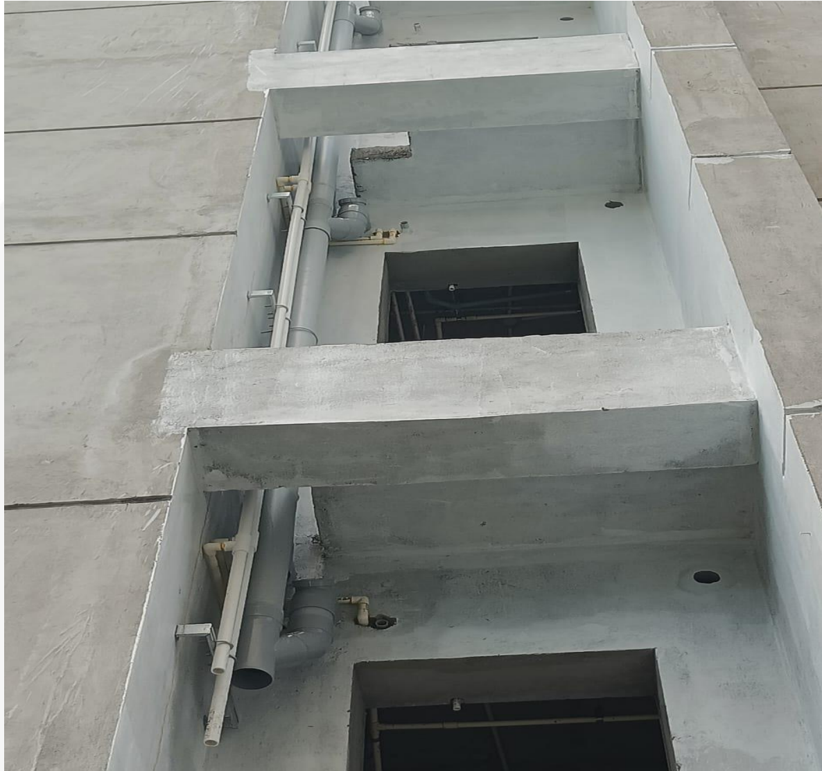
Wing 3D, External Shaft - Plumbing Works in Progress
