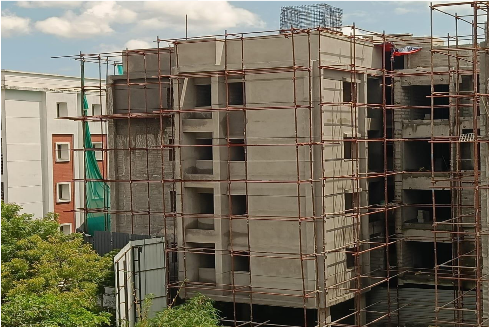
Wing 3B – North Elevation View
