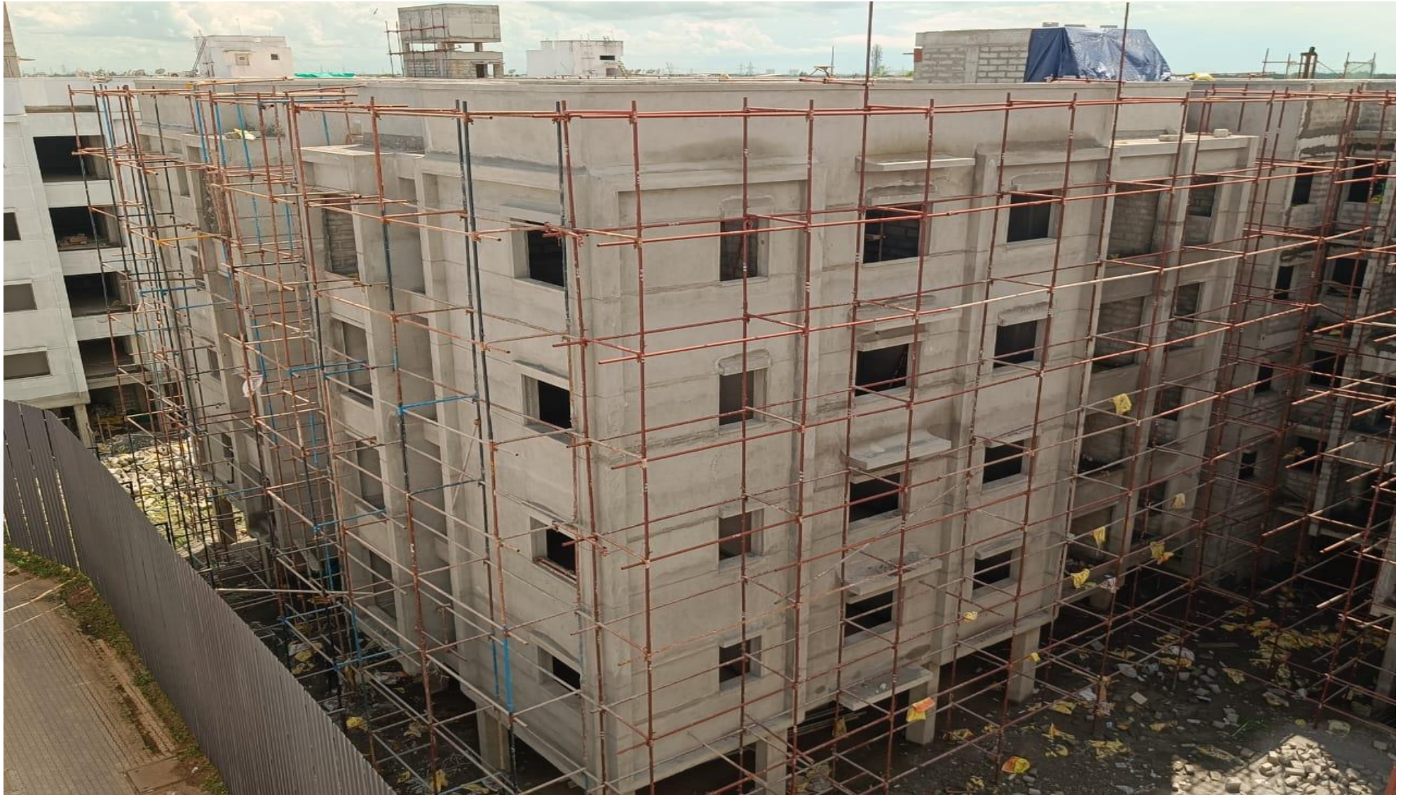
Wing 3C – North & East Elevation View
