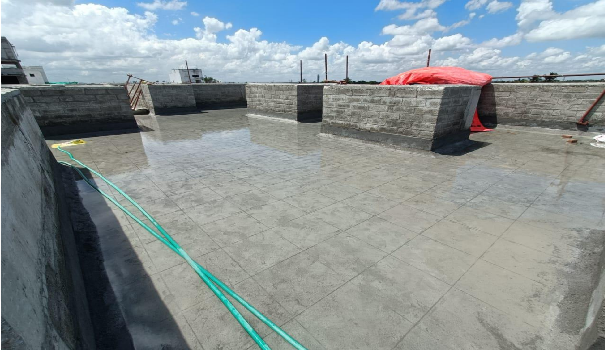
Wing 3C, Terrace - Water Proofing Works in Progress
