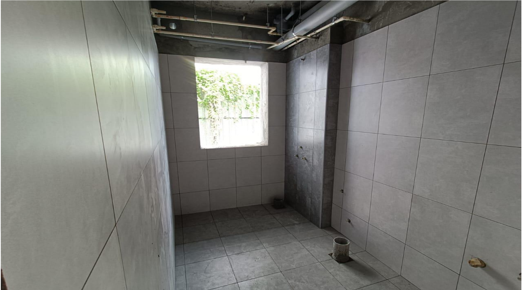
Wing 3D, 1 st Floor – Toilet Tile Works in Progress
