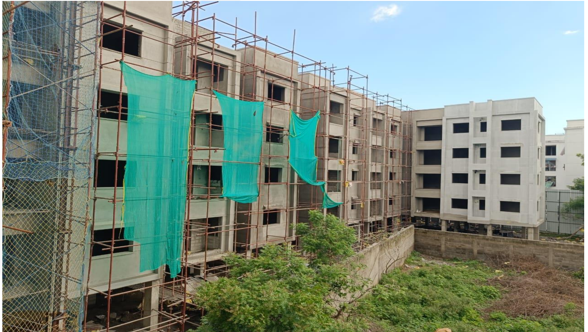
Wing 3C & 3E – West Elevation View
