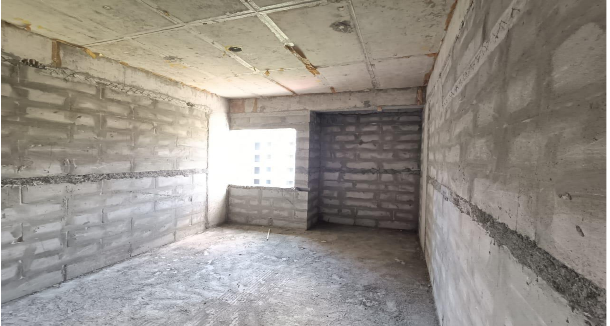
Wing 4A & 4B , 3 rd Floor - Block work in progress
