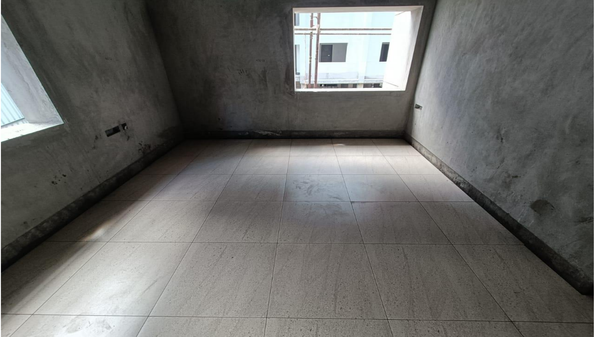
Wing 3E, 1 st Floor - Tile Flooring Works in Progress
