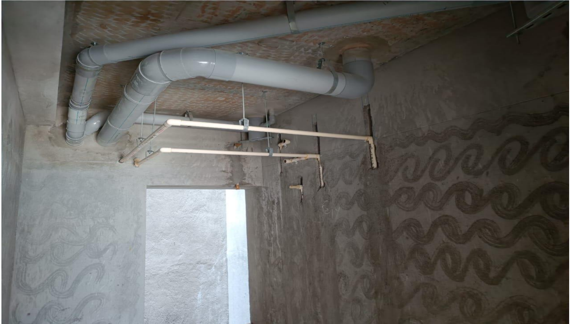
Wing 3C– Toilet’s Ceiling Suspended Line Works in Progress
