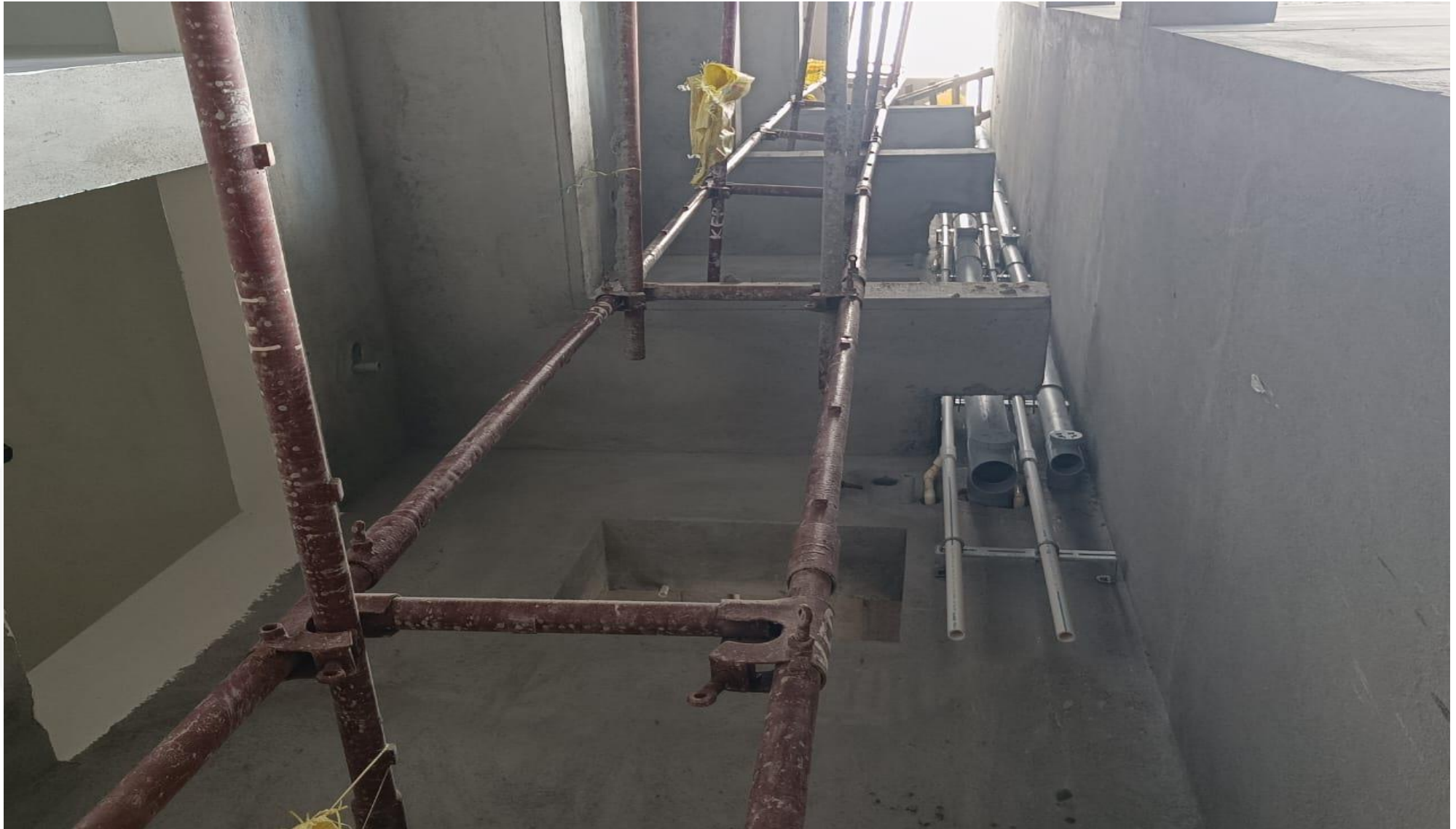
Wing 3D, Toilet Shaft - Plumbing Works in Progress
