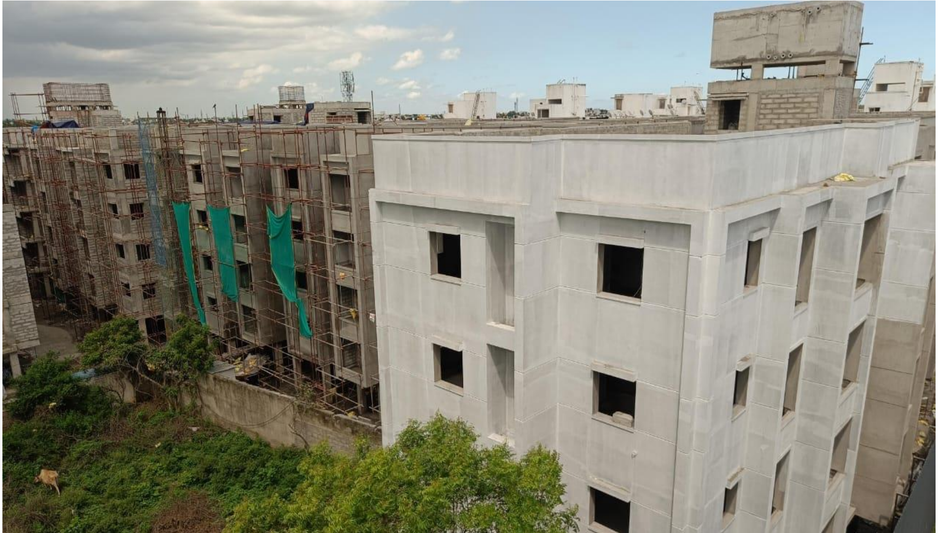
Wing 3E, 3C & 3A – West Elevation View
